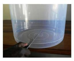
This can be done by hand with a sharp tool or knife. Make a hole just big enough to tightly fit the back of the tap, which is approximately 12,5cm in width, into it. Make the hole about 4cm above the bottom of the bucket/water storage vessel. This height will prevent settled sediment from entering the filter/purifier.
